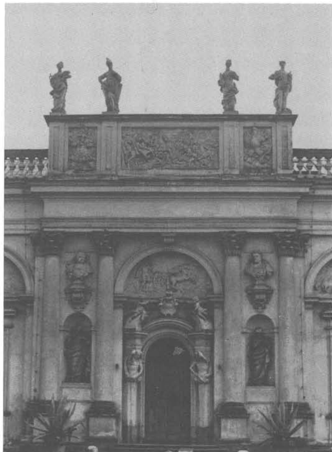
18. The Palace of Wilanów. Front elevation of southern wing (detail) showing reconstructed statues of attic
